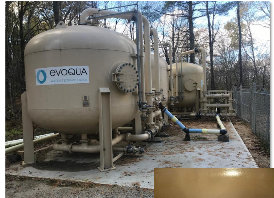
Right | Interior lining of GAC vessel with Septa underdrain design
