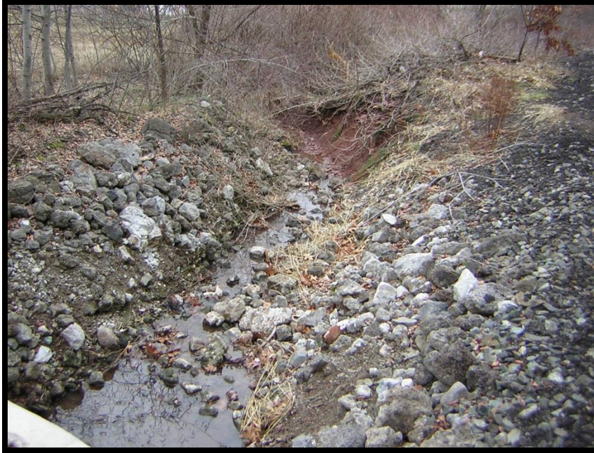
Manmade Channel in Poor Condition
